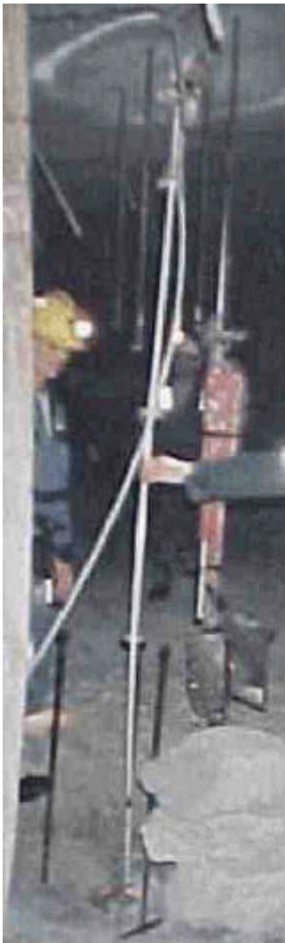
Figure 7. Contractometer installation prior to forming and shotcrete placement.
