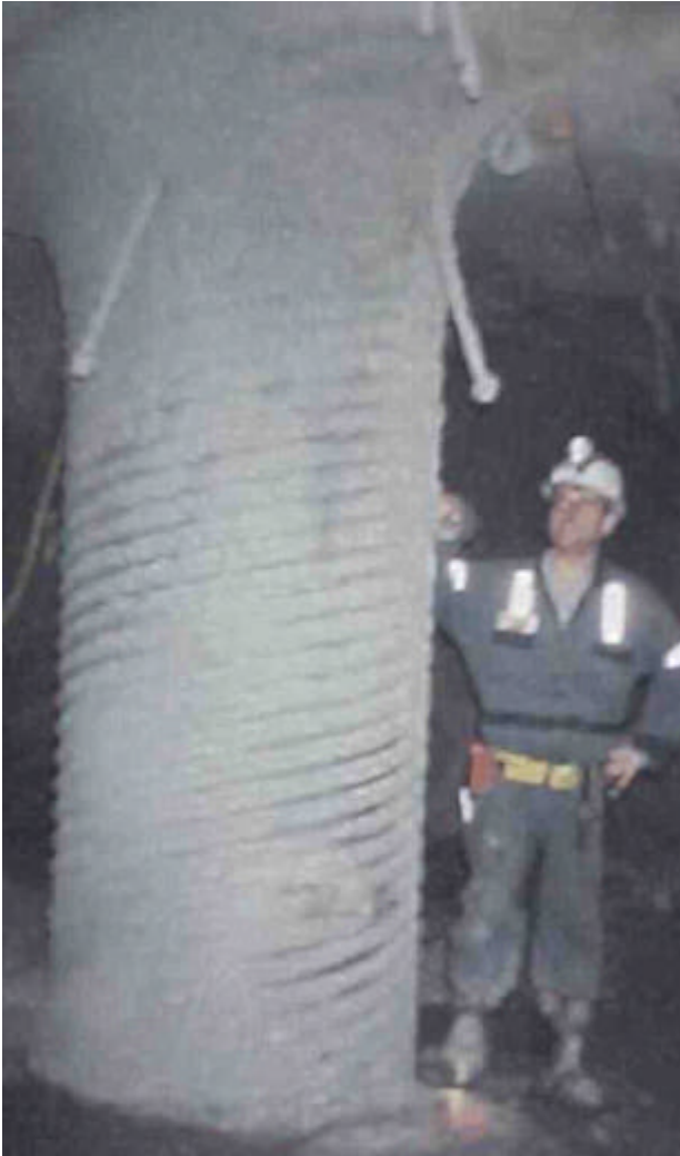
Figure 6. Completed shotcrete pillar.
